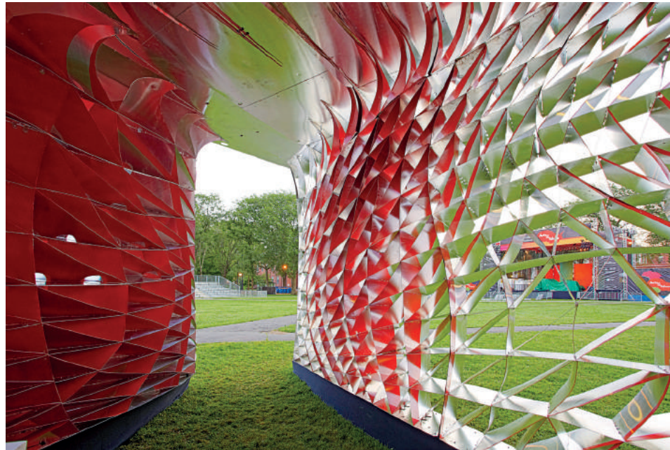
Fig. 4: Constructed from thin aluminium sheets, the pavilion opens up on two sides for ventilation and security, focusing the view toward the festival's main stage. (Photo: Chris Morgan Photography.)
