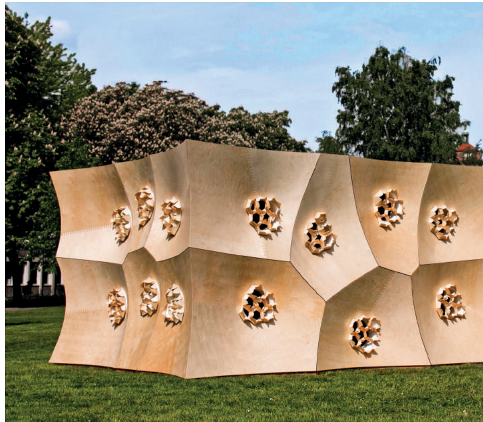
Fig. 12: Photo of the HygroSkin – Meteorosensitive Pavilion in Stadtgarten, Stuttgart. Low relative humidity, 45%, with open HygroSkin surface.
