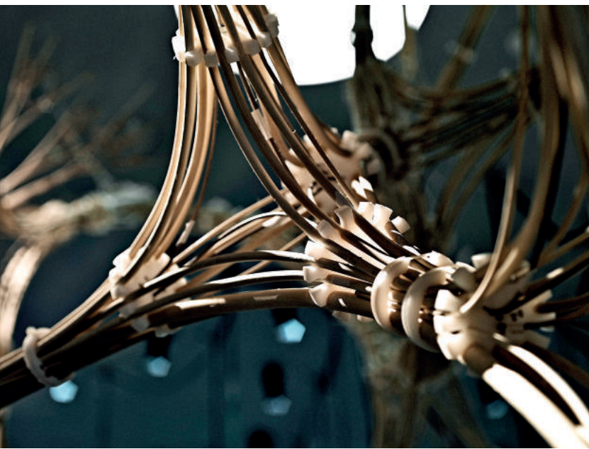
Fig. 12: Star nodes for organising oppositional active-bending rattan branch connection elements for both structural performance and bespoke geometric deployment with inner grey guideposts.
