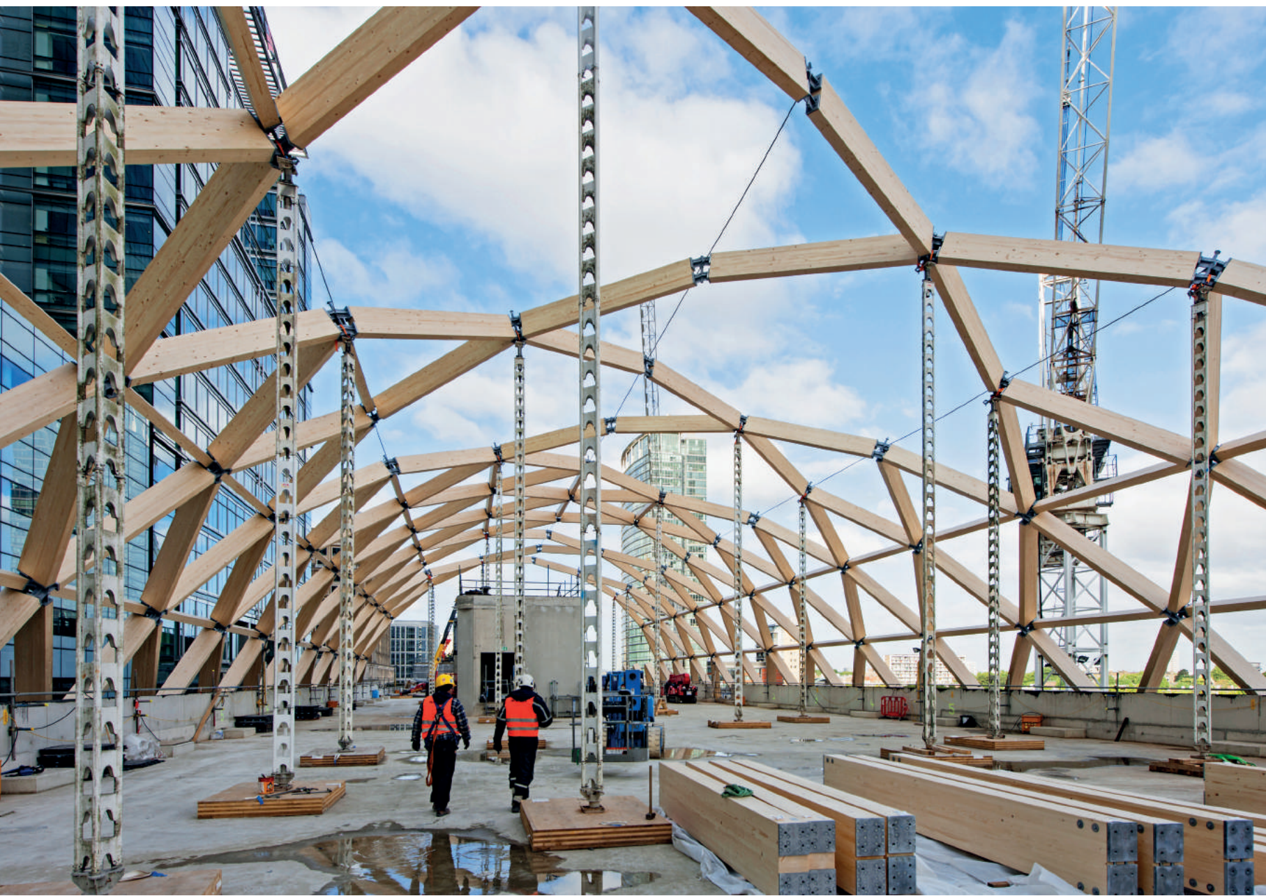
Fig. 1: Photograph showing timber grid shell structure over the central third of the roof. Construction progress mid November 2013. (Photo: Nigel Young / Foster + Partners.)
