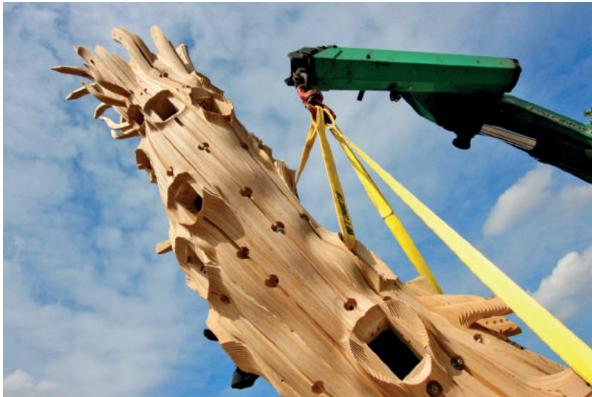
Fig. 5: Assembled, denuded trunk core being lifted for transport to first site.
