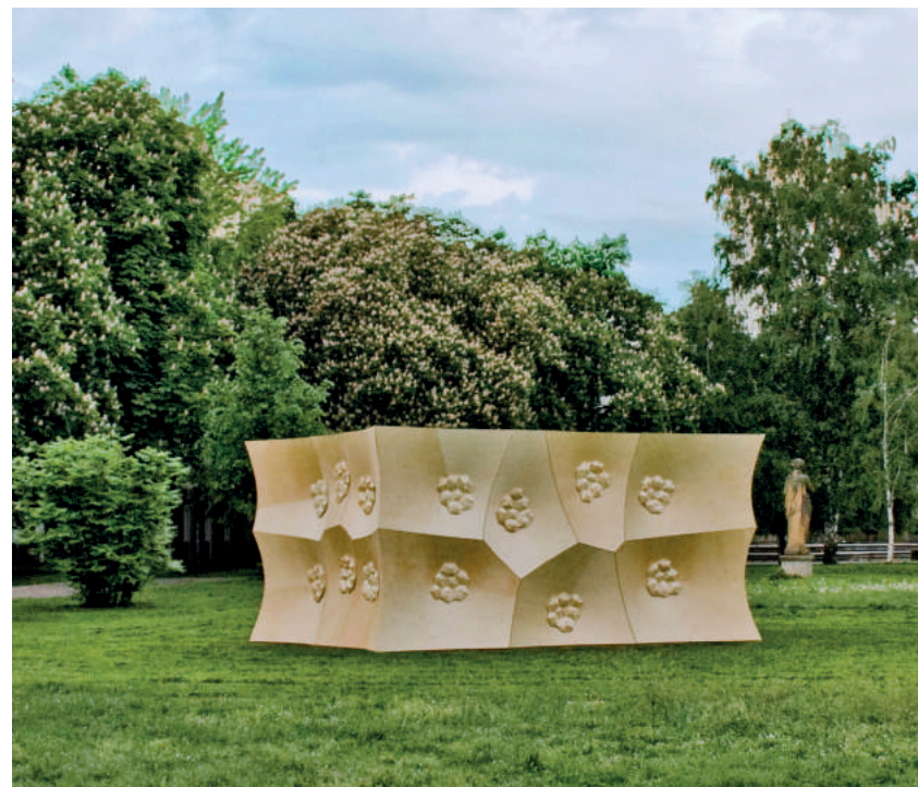
Fig. 2: Photo of the HygroSkin – Meteorosensitive Pavilion in Stadtgarten, Stuttgart (high relative humidity, 75%).
