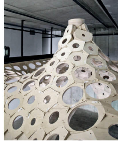
Fig. 4: The upper bound geometry skips continuity at the connection of the voussoirs due to the requirement for the milling operation to have a flat surface.
