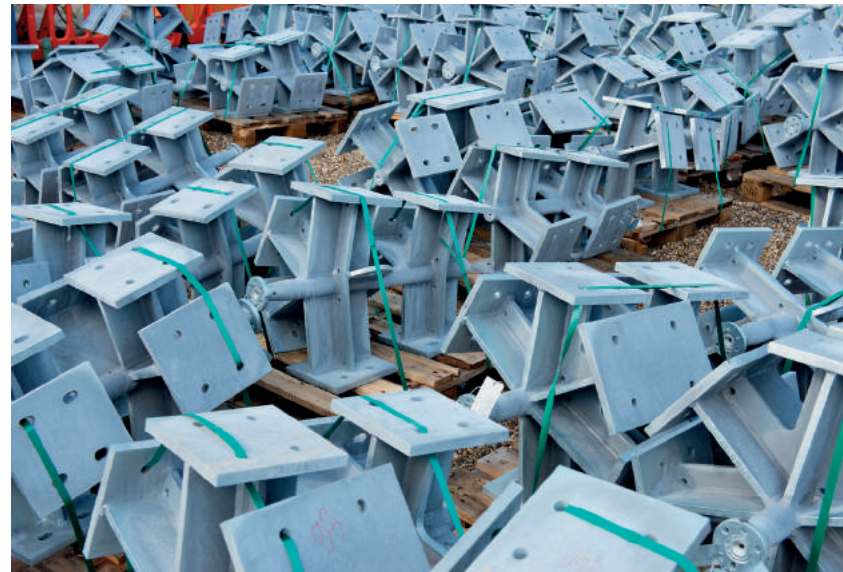
Fig. 9: Photograph capturing an array of nodes stored on site awaiting installation. Clearly seen is the differentiation of node geometry and variation in number of connection arms. (Photo: Nigel Young / Foster + Partners.)
