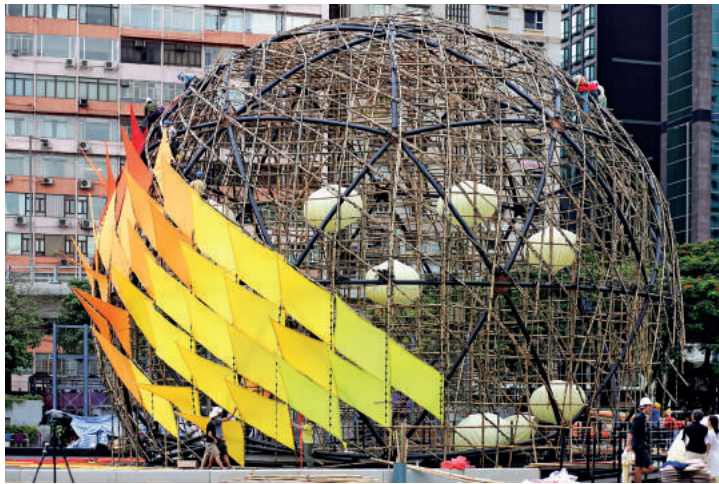
Fig. 7: Installation of stretch fabric flames. (Photo: Kevin Ng.)
