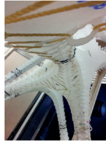
Fig. 11: Nylon string laced through tabs in plastic formwork.
