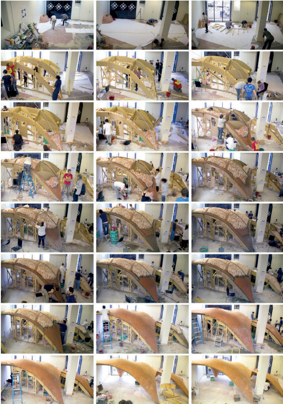
Fig. 7: Construction time lapse of MADA vault. (Photo: Dean Lau Tim Ling.)
