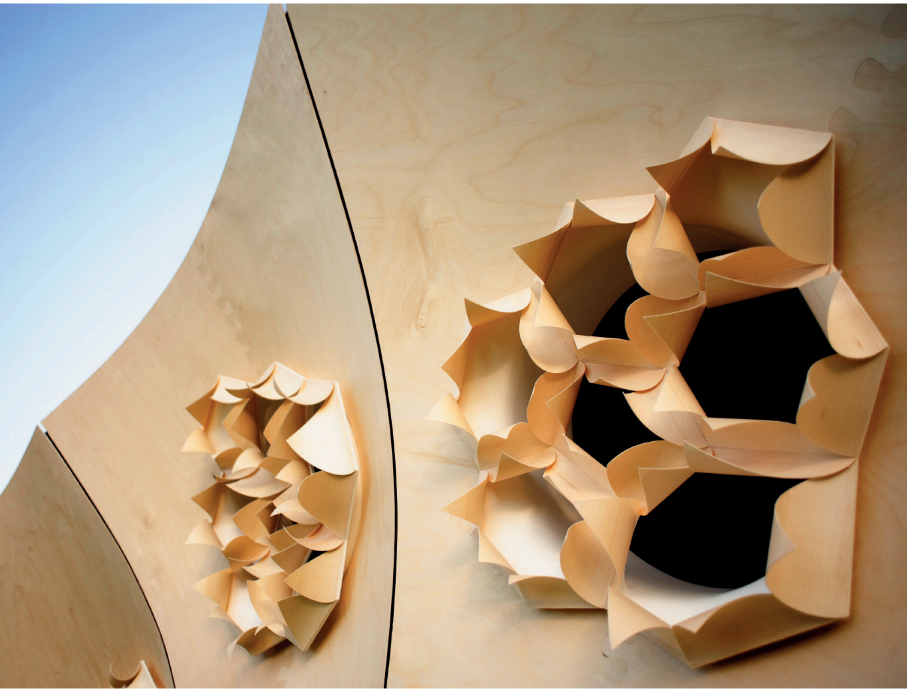
Fig. 1: Close-up photo of the HygroSkin – Meteorosensitive Pavilion (low relative humidity, 45%).
