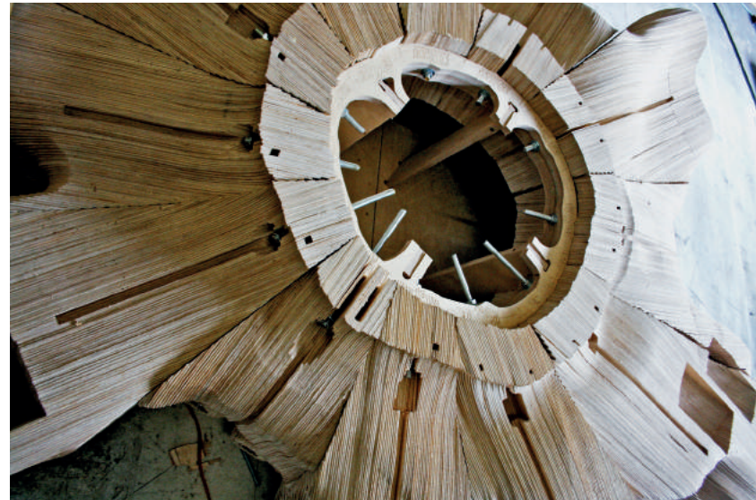
Fig. 6: View past lowest tree ring into the void of the trunk base, without ballast.
