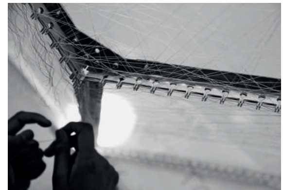
Fig. 10: Knotting of vertex connections of non-woven silk patches on temporary aluminium scaffolding structure.
