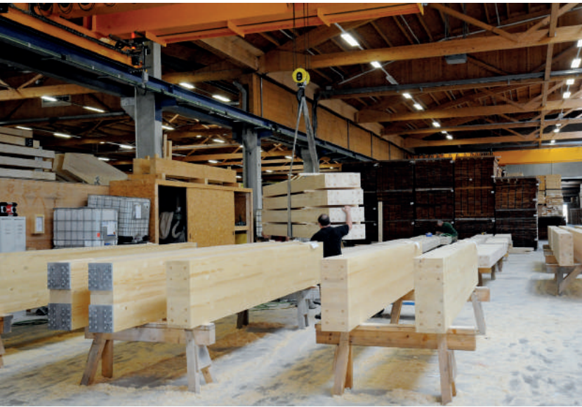
Fig. 6: Photograph showing machined glulam beams awaiting attachment of end plates. This process involves screwing in timber screws using a hand-held drill. Stacked in the background are timber planks that have arrived directly from the sawmill. Wiehag Factory, Altheim, Austria. (Photo: Mitterbauer.)
