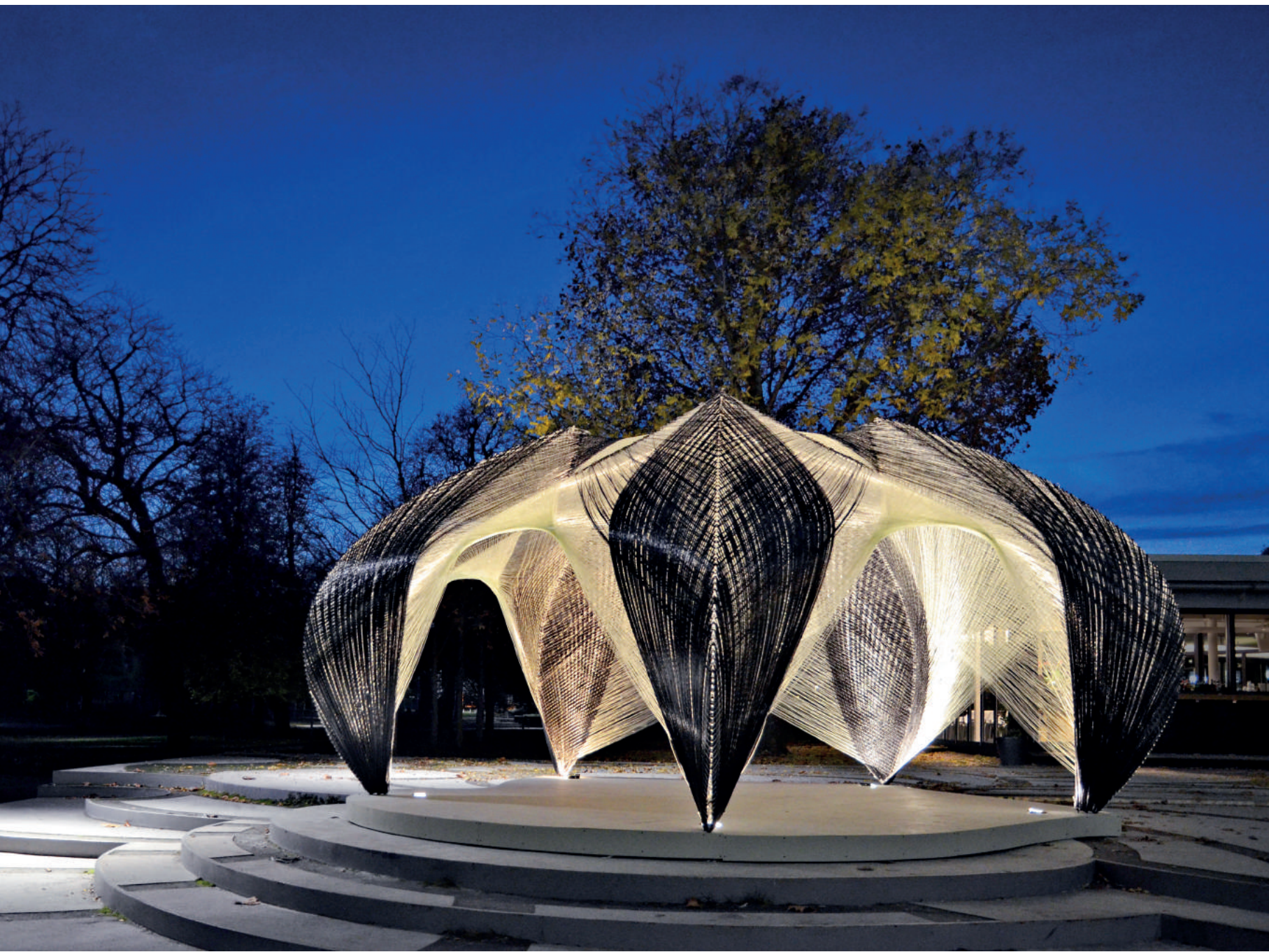
Figs. 2, 3: Institute for Computational Design, Institute of Building Structures & Structural Design, Faculty of Architecture and Urban Planning, University of Stuttgart, ICD/ITKE Research Pavillion, final installation, Stuttgart, 2012.
