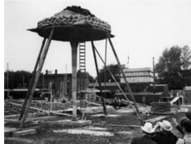
Fig. 1.4 Frank Lloyd Wright witnessing the load testing a prototype concrete column for the Johnson Wax Administration Building
