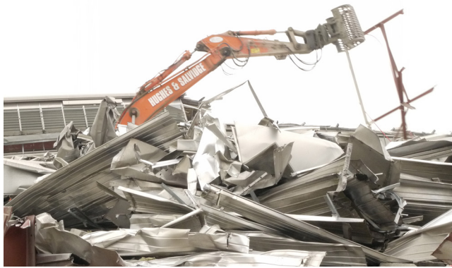
Fig 8.20 Sadly the demolition and recycling of Chetwoods Architects' award winning North Greenwich Sainsbury's was predicted in TSC Book Two Aluminium Recyclability and Recycling , demolition took place in the spring of 2016. An over 99% recycling rate of steel and aluminium was recorded on site by contractors Hughes & Salvidge
