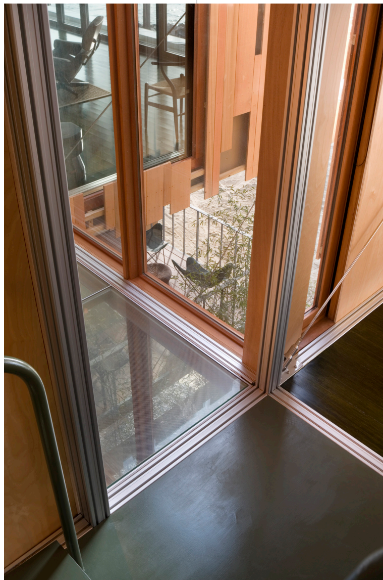
Fig 3.7 The extruded aluminium frame of the Loblolly House, Maryland, USA. Architect KieranTimberlake, 2006
