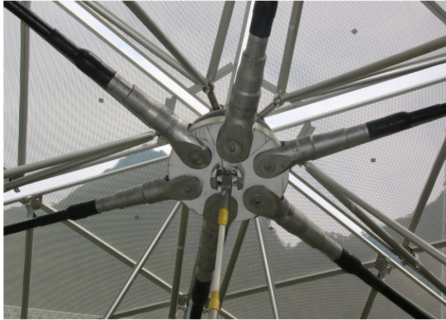
Fig 8.2 Detail of the assembly of The Five Hundred Meter Aperture Spherical Radio Telescope, which is clad in perforated aluminium
