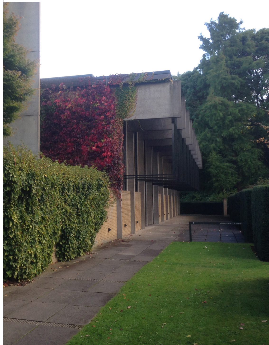
Fig 6.75 Aluminium solar shading of the Grade 1 listed – St Catherine's College, Oxford, England, architect Arne Jacobson, 1964, photographed in 2016
