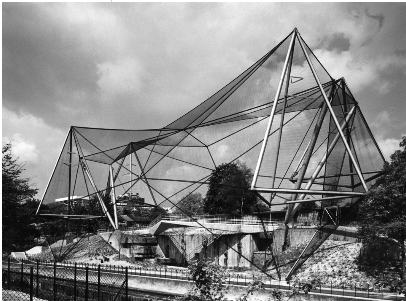
Fig 8.35 The Snowdon Aviary, with its tubular aluminium alloy structure, at London Zoo, architect Cedric Price with engineer Frank Newbery and detailed input from Lord Snowdon, completed in 1965. The Snowdon Aviary is Grade II* listed by Historic England (13223695). In 2017 Foster + Partners are in the process of restoring this enclosure and converting to house Colobus monkeys
