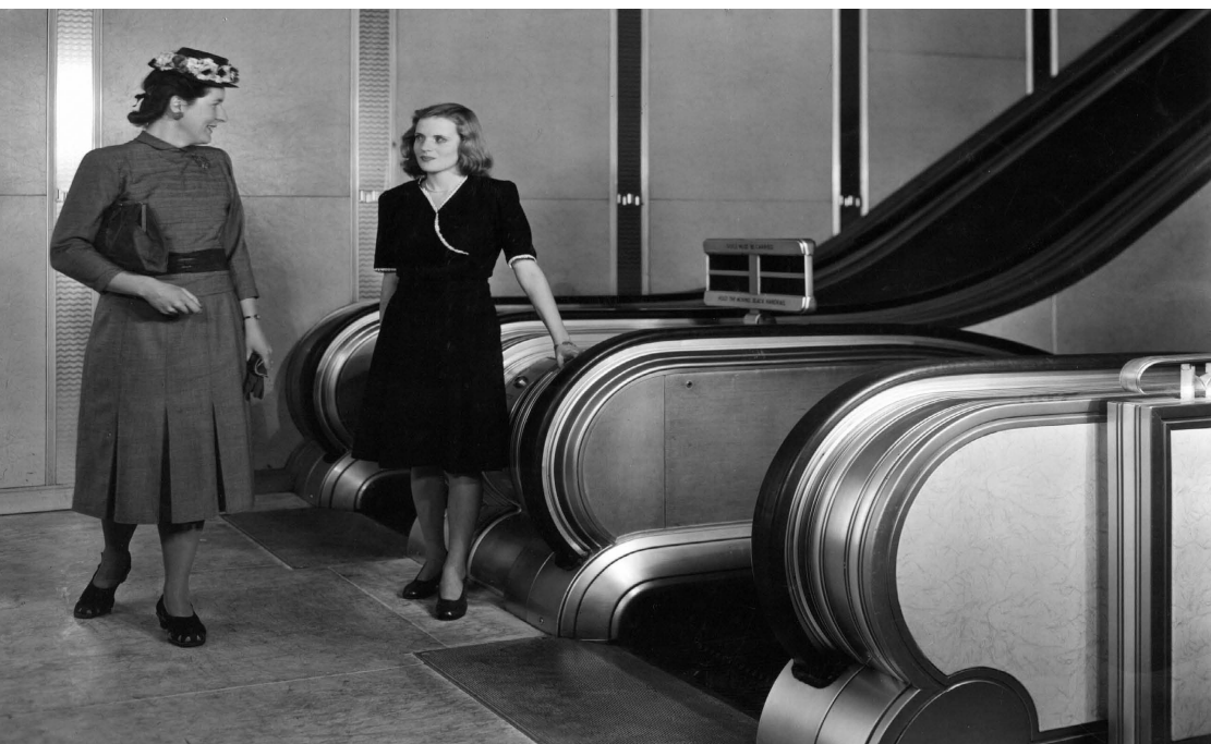
Fig 6.11 Detail of the curved and profiled aluminium escalator cladding
