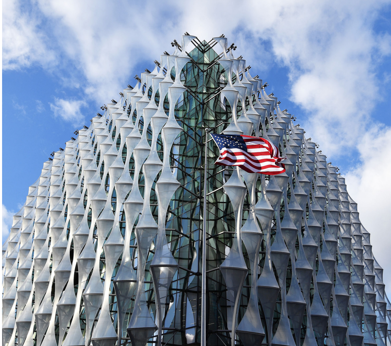
Fig 8.33 ETFE solar shading on aluminium armatures, the new American Embassy, London, England, architect KieranTimberlake, 2018
