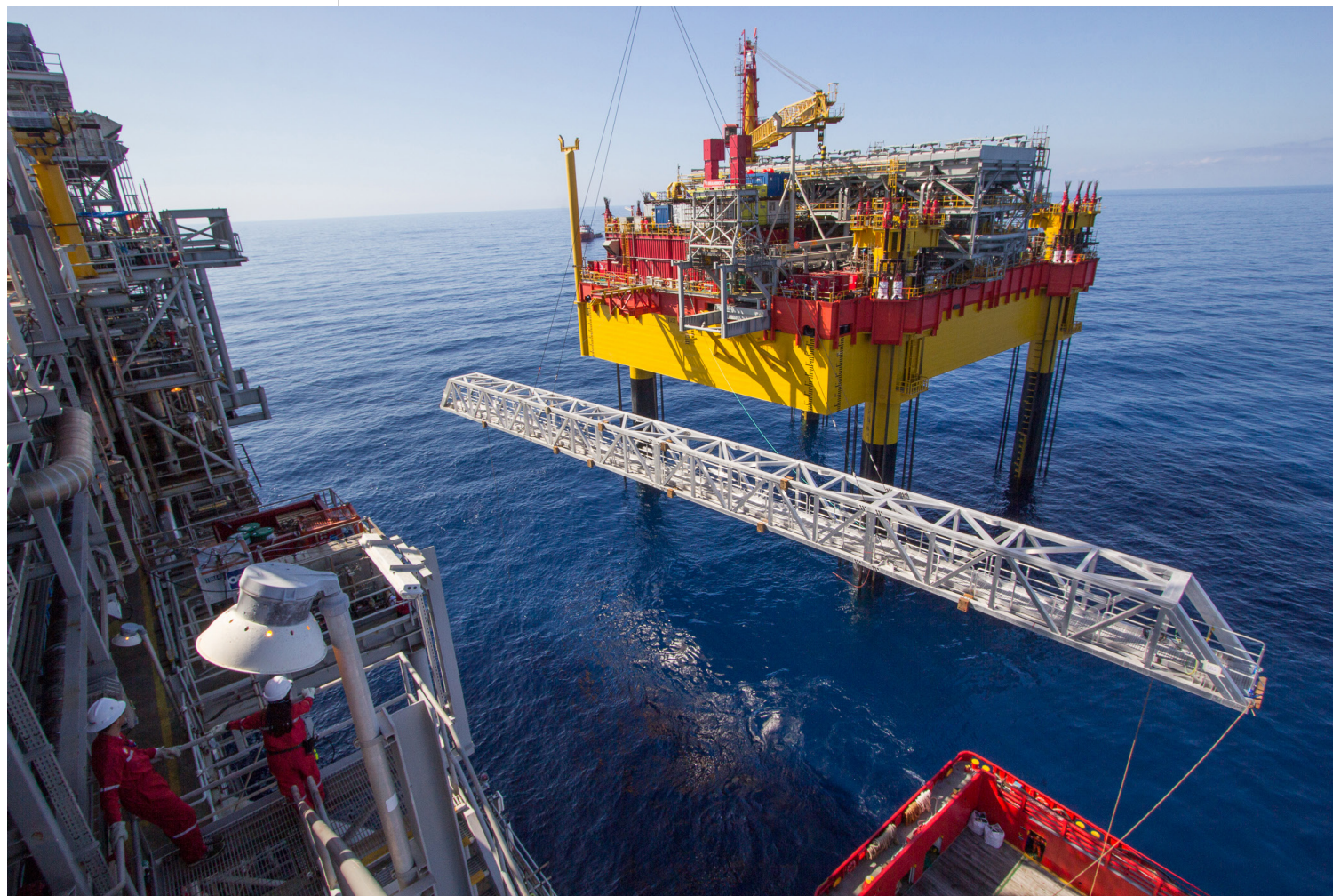
Fig 5.21 46,3m welded aluminium alloy bridge, designed and fabricated by MAADI, being craned into position, 2014, published with permission from the oil extraction company
