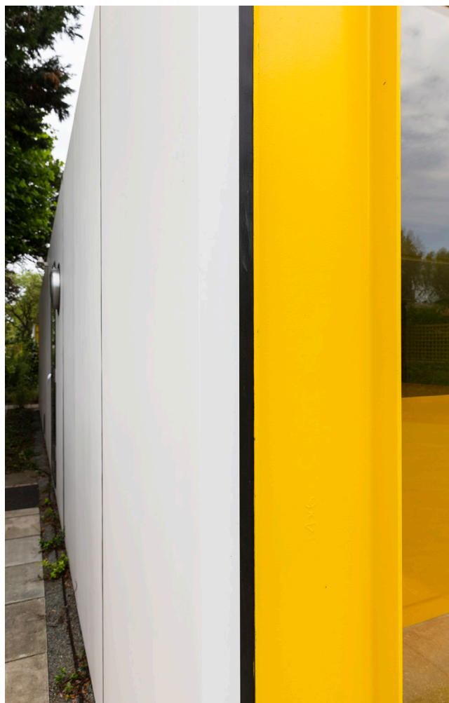
Fig 6.28 Rogers House, 2017, detail of the polyester powder coated aluminium wall panel meeting the painted steel portal frame
