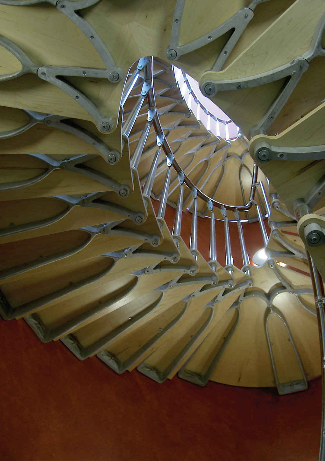
Fig 8.22 Cast aluminium and maple stair in Tudor House, architect Knox Bhavan, 2003
