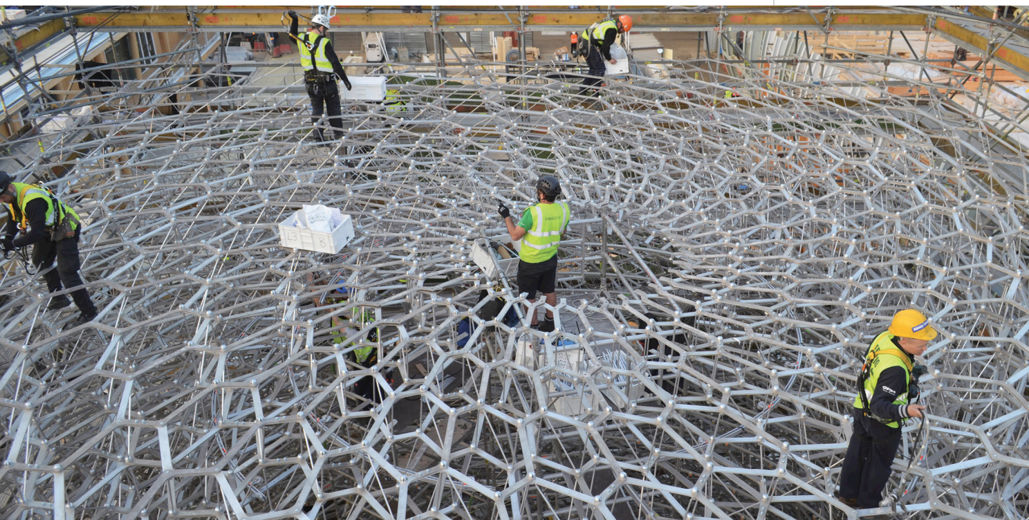
Fig 2.3 The aluminium meshwork of the Hive being assembled by Stage One in Milan, 2015
